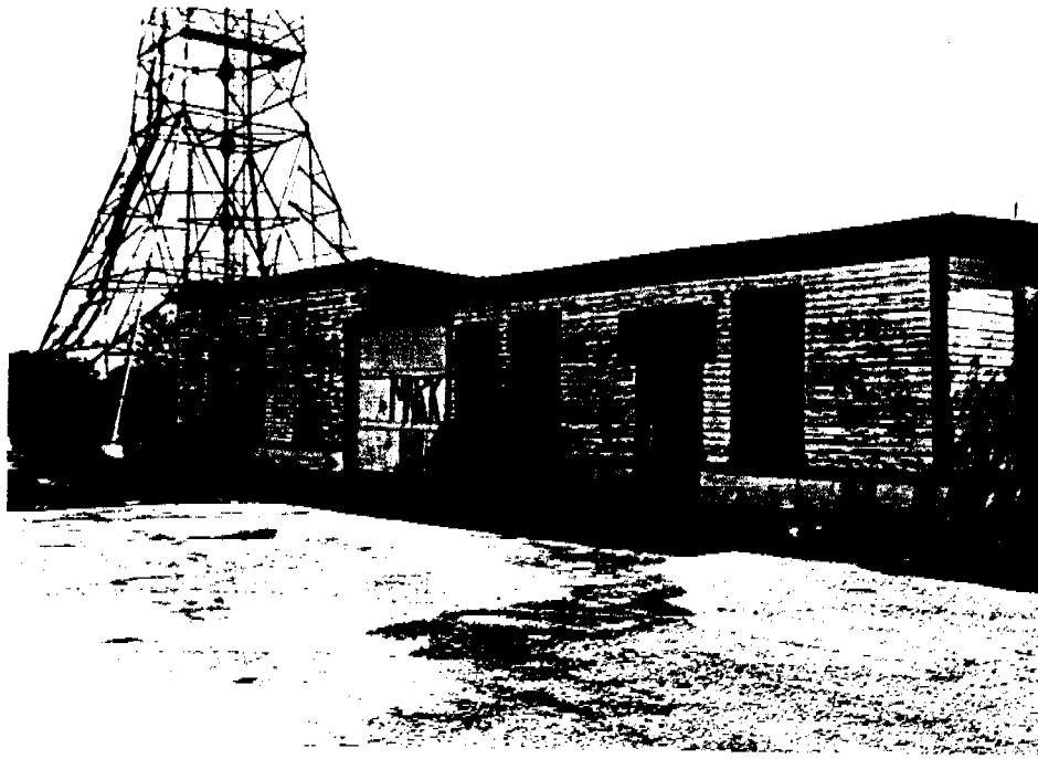
Neg. KK XXV-7, fm. SW, showing base of FAA tower and clapboard building with a brick foundation east of the power house.
