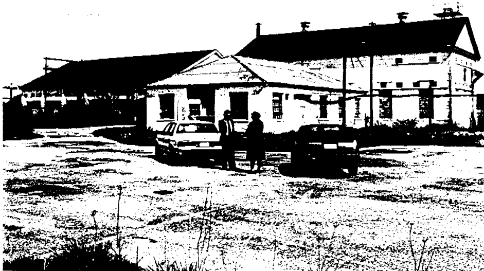
Neg. KK XXV-12, fm. SE, showing power house and smaller hip roof building. The two large gable roof concrete buildings in the background are connected by a one-story link.
