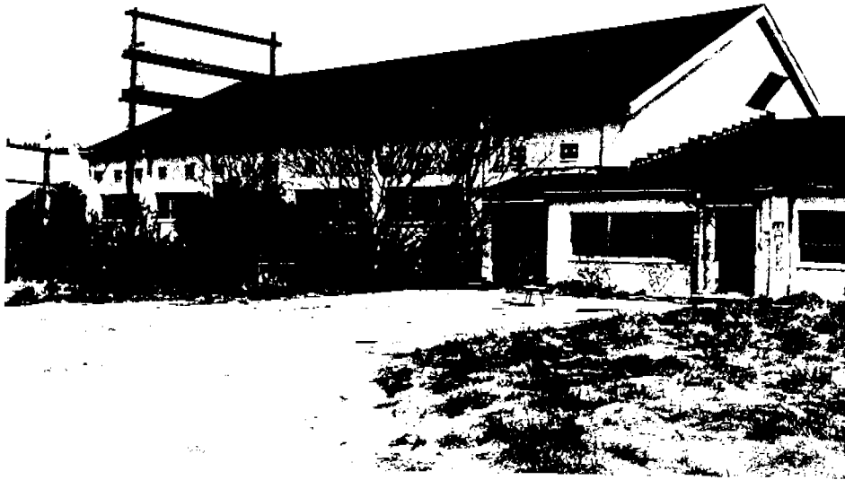
Neg. KK XXV-8, fm. SE, showing west wing of power house.
