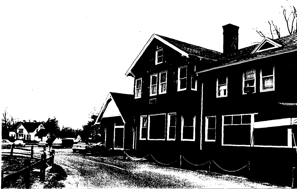
Neg. KK VI-6, fm. S/SW. View of original overhanging gable at far left.
