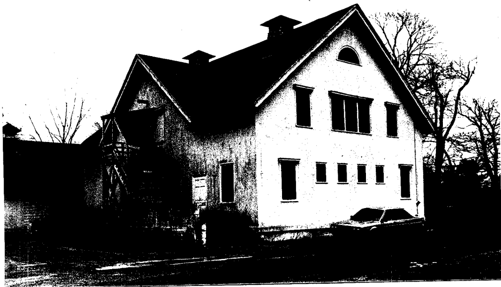
Neg. KK VI-17, fm. W/NW. Barn, north and west facades.
