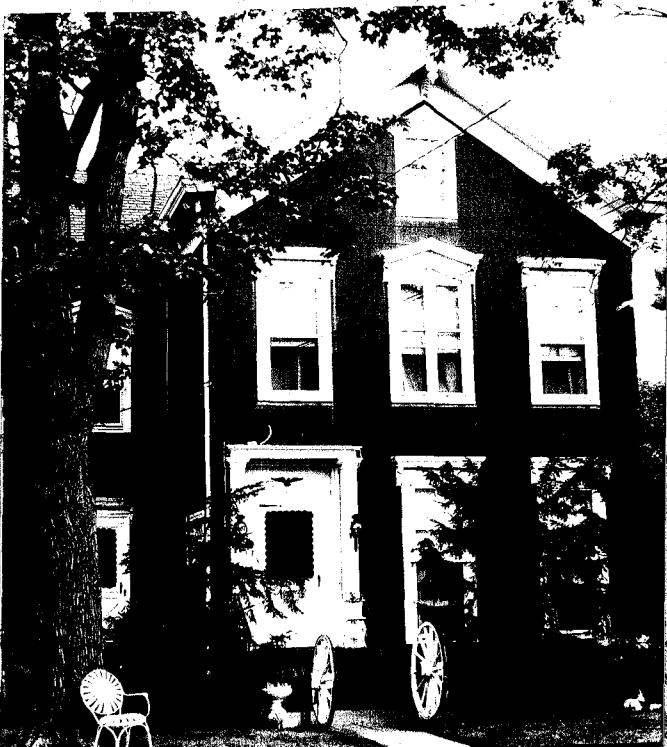
Day Shore Roll #Q4; Neg. #18 HP-1 Front (west) facade.
