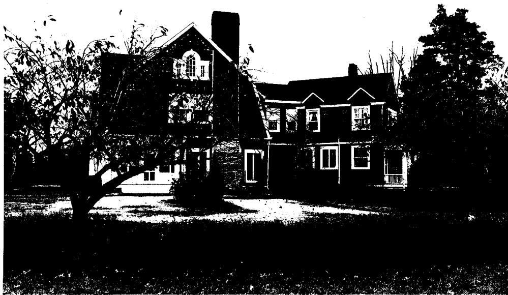
Neg. KK I-21, fm. SE. East chimney and angled wing.
