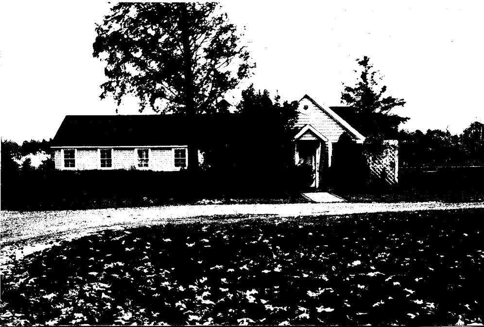
Neg. KK I-36A, fm. W. Outbuildings remaining from the Pinkerton estate.
