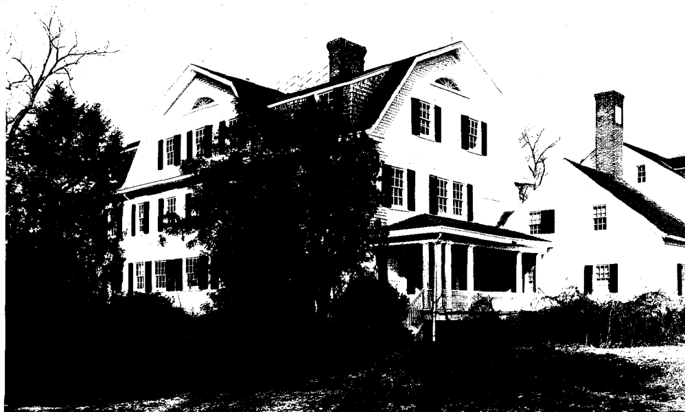
Neg. KK VIII-5, fm. SW, view of wing designed by I.H. Green.
