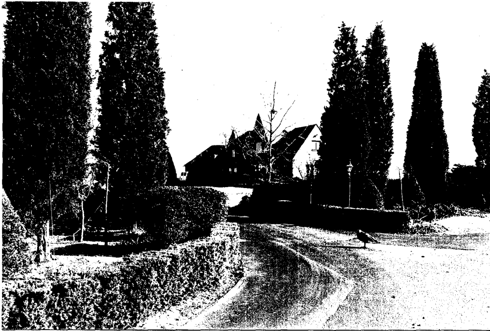
Neg. KK V-13, fm. NW, showing driveway entrance to Entenmann House from the end of Lawrance Lane at the peninsula point.
