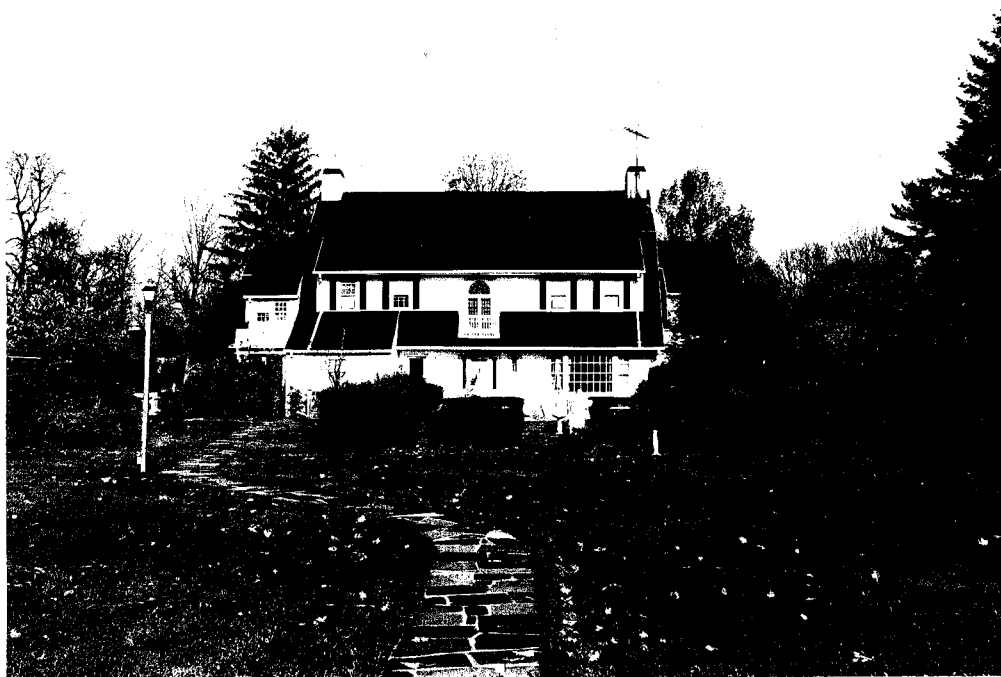
Neg. KK IV-7, fm. west, garden facade.
