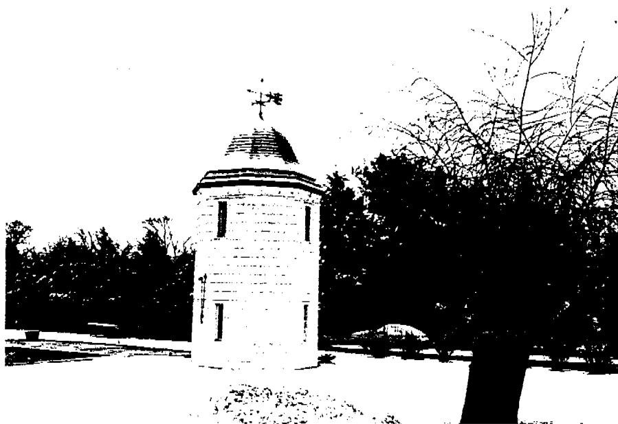
Neg. KK XX-10, fm. NE, view of tower from stable wing in photo below.
