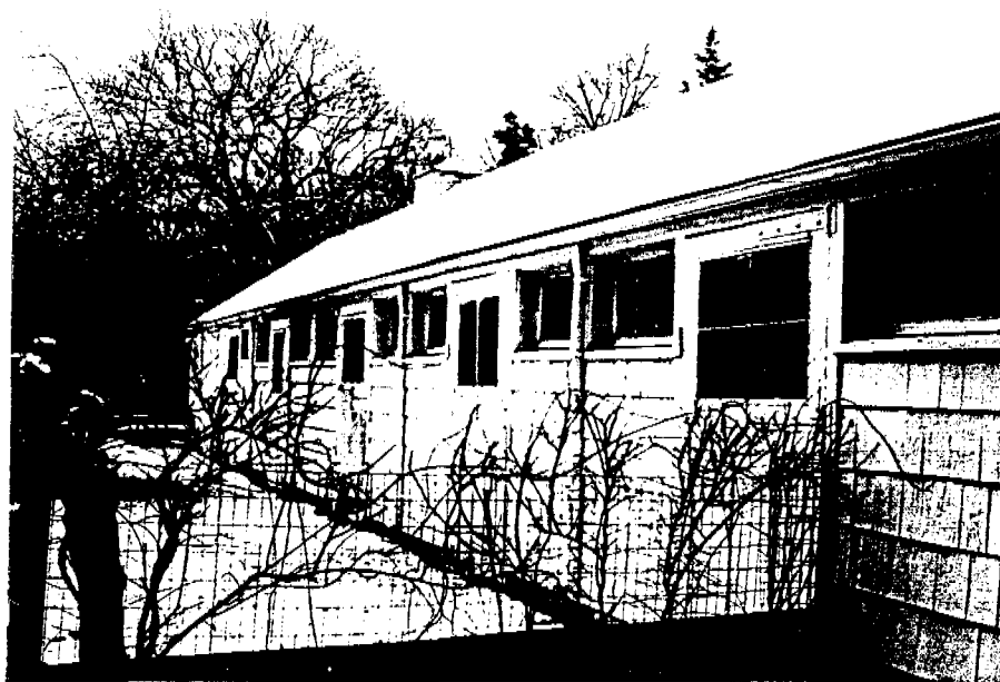
Neg. KK XX-8, fm. N/NE, view of stable wing from greenhouse yard.
