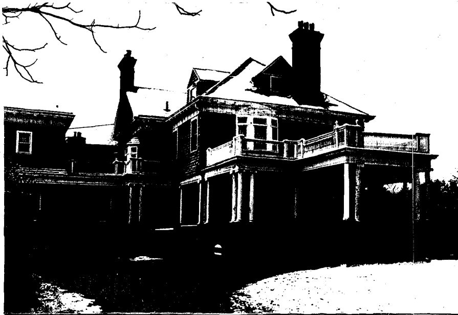
Neg. KK XX-17, fm. N/NE, showing a section of the east wing.
