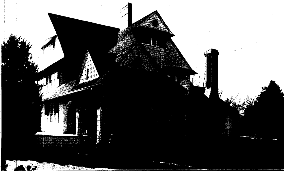
Neg. KK III-5. J. Mollenhauer House, detail of porte cochere from NE.
