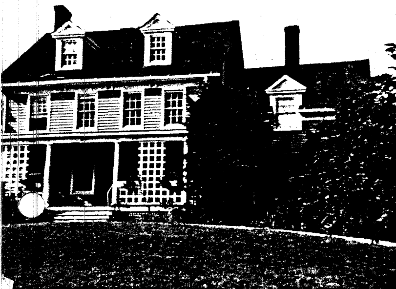
Ockers House, prior to fire. (c.1978)
