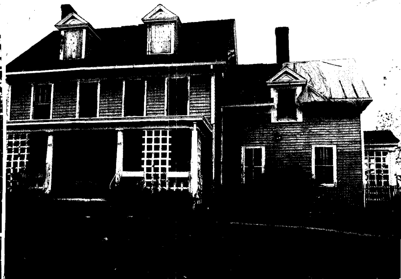
Ockers House, after fire. (1991)
