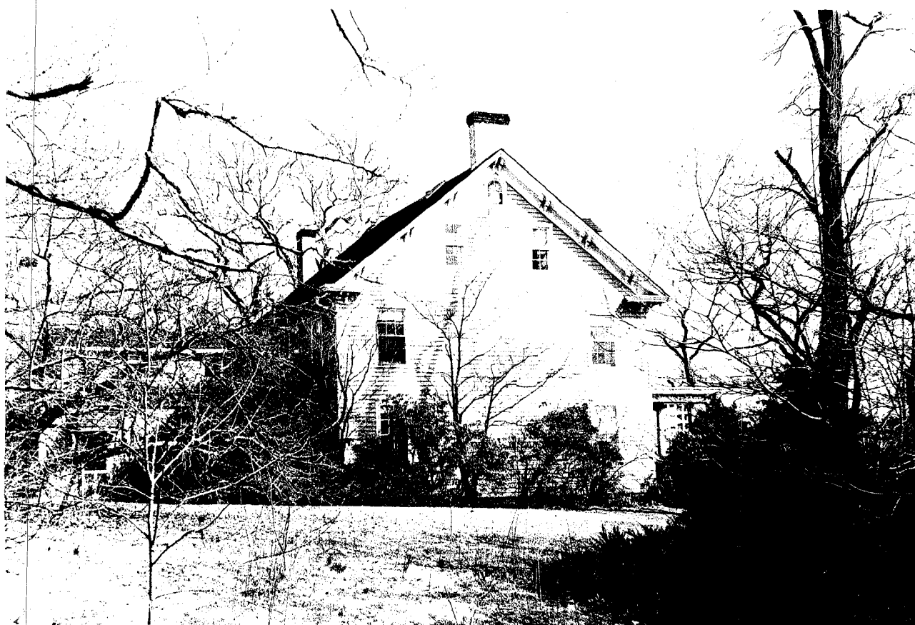
The west side of the house
