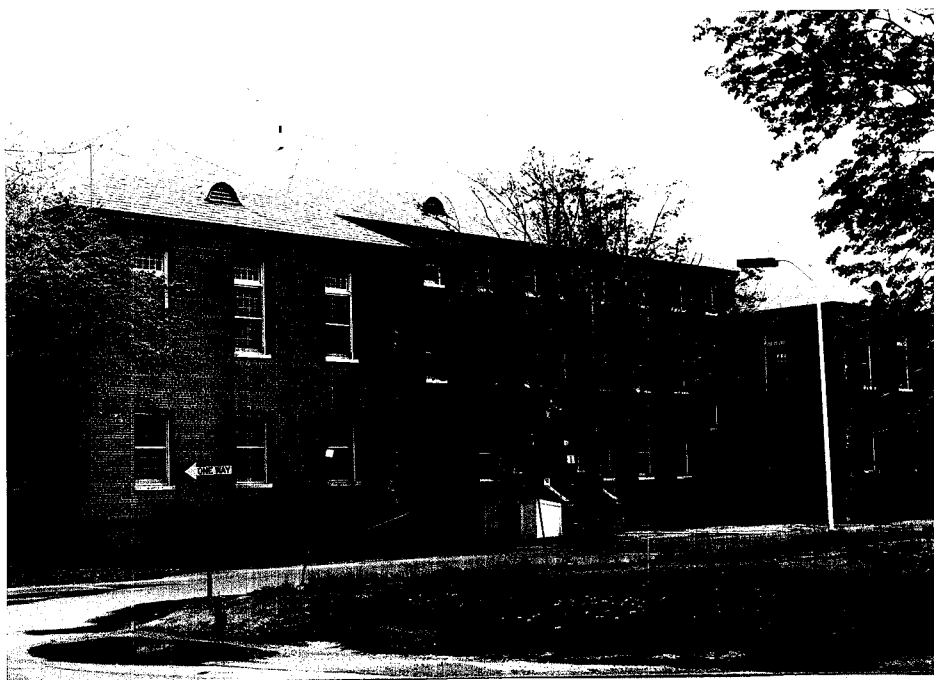
Building L-1 Photo:CI-WHC-r-1,28 from SE
