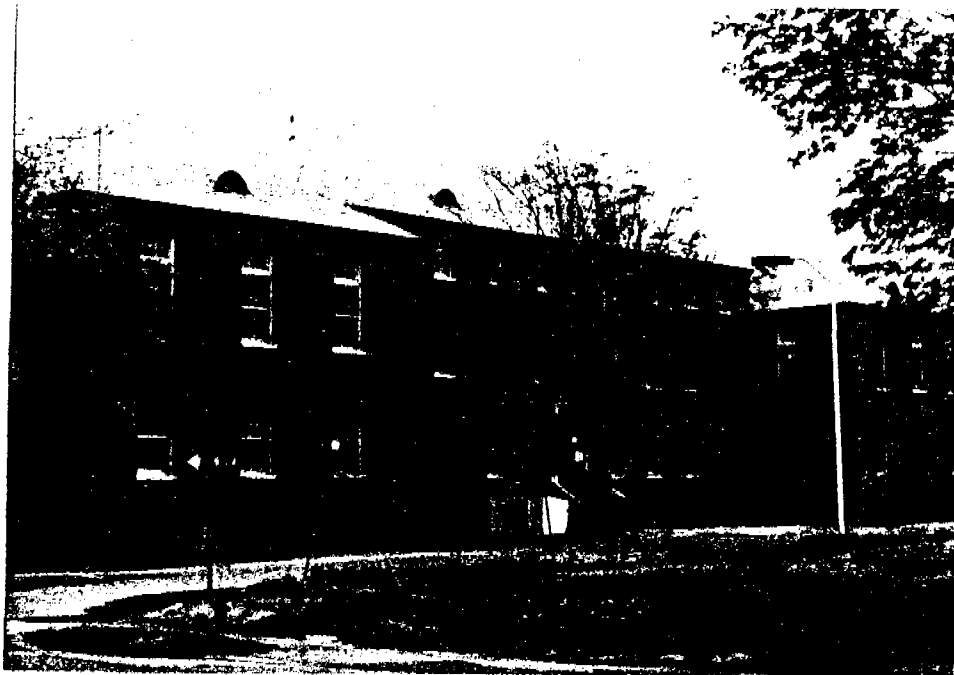
Building L-1 Photo:CI-WHC-r-1,28 from SE
