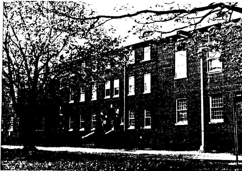
Building L-5 Photo:CI-WHC-r-1,22 from SE
