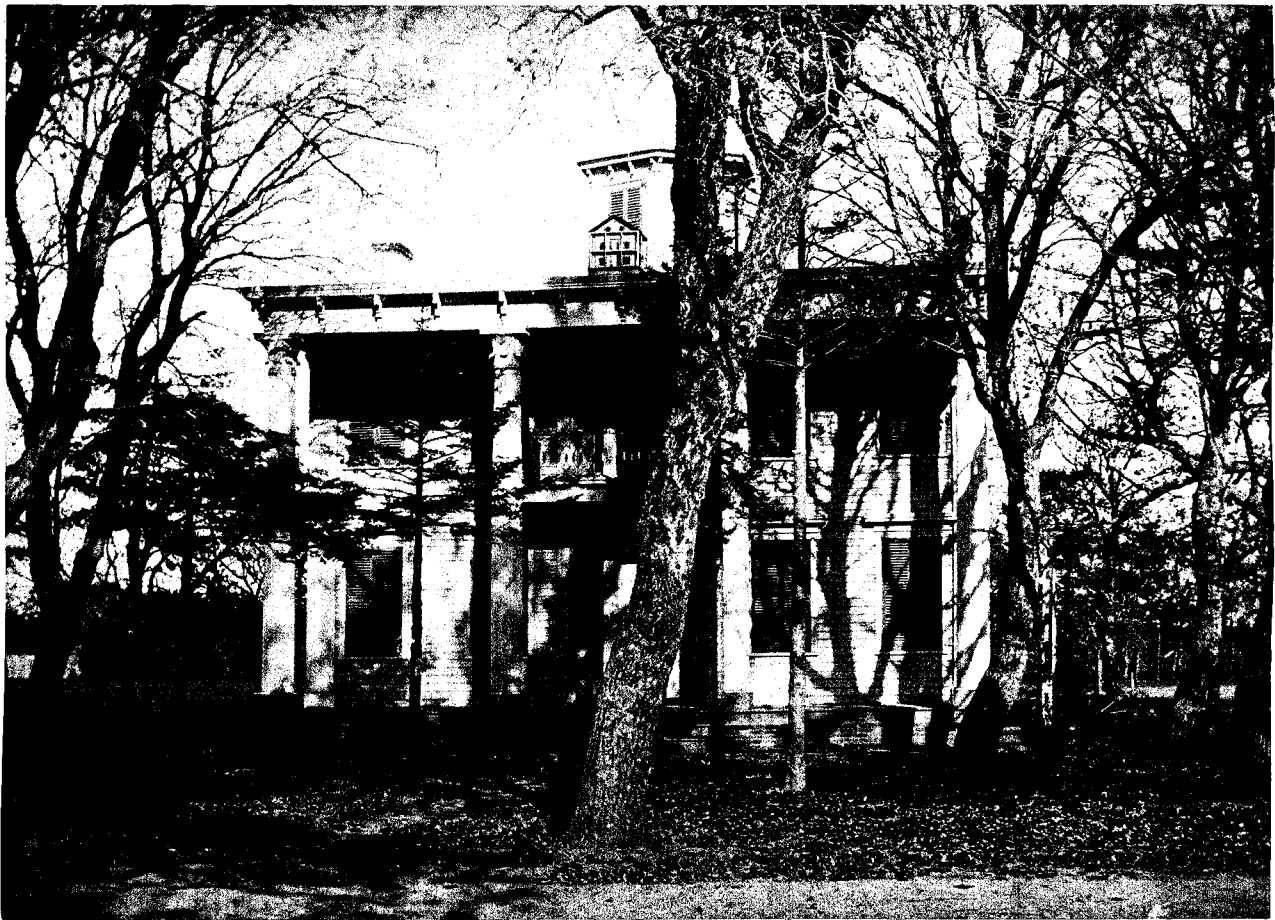
1885 view, front (from south)
